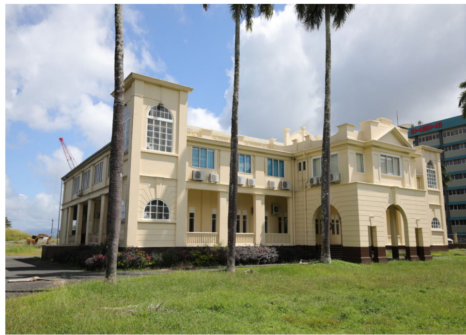
Cabinet approved the second development phase for the establishment of St. Stephen's building as Fiji's first National Art Gallery. Photo: AZARIA FAREEN
