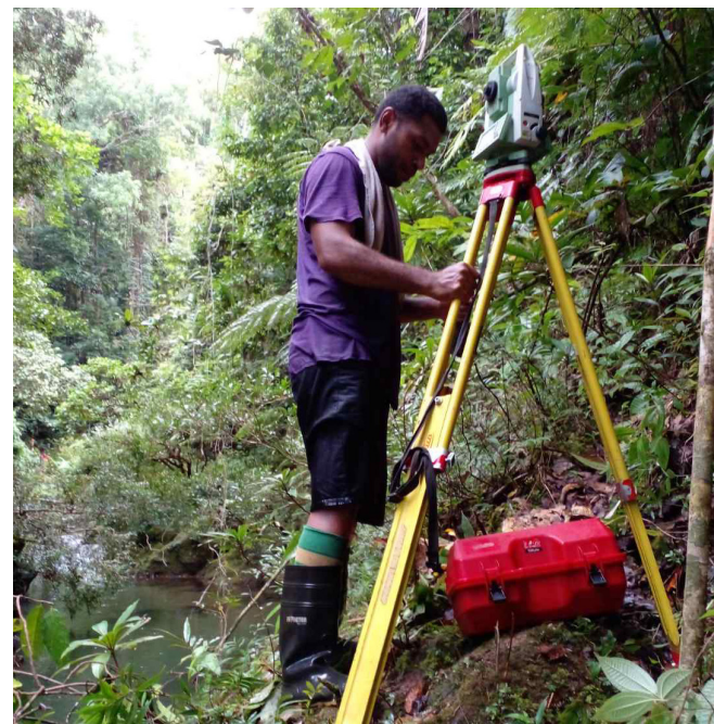
A surveyor at work with a Theodolite. Photo: SUPPLIED
