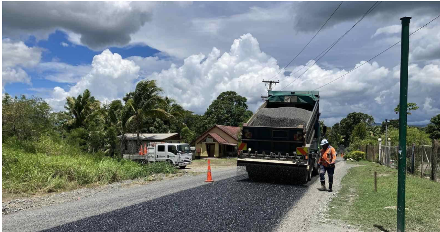
The sealing of Legalega Road in Nadi has been completed, along with drainage improvement works. A total of 650 meters has been sealed, providing safer, and more reliable access for daily commuters, school children, and nearby residents. Minister for Public Works, Meteorological Services & Transport, Filipe Tuisawau, highlighted that infrastructure development is not just about roads and bridges, but about “progress that touches every Fijian household”. Photo: SUPPLIED
