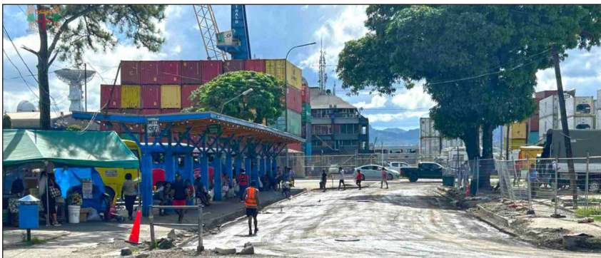
Fiji Roads Authority (FRA), in collaboration with the Suva City Council, is currently undertaking much-needed pavement works at the Suva Bus Stand. Photo: SUPPLIED
