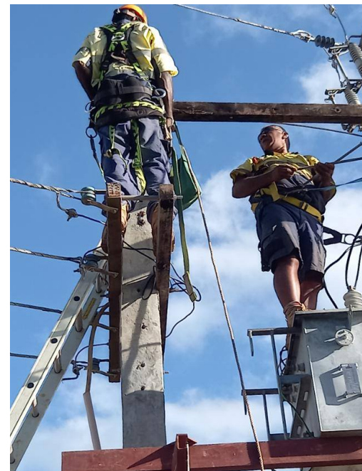
The Electrical Division of the Public Works Department is conducting repair and maintenance work on the grid in Vunisea, Kadavu Island . Photo: SUPPLIED
