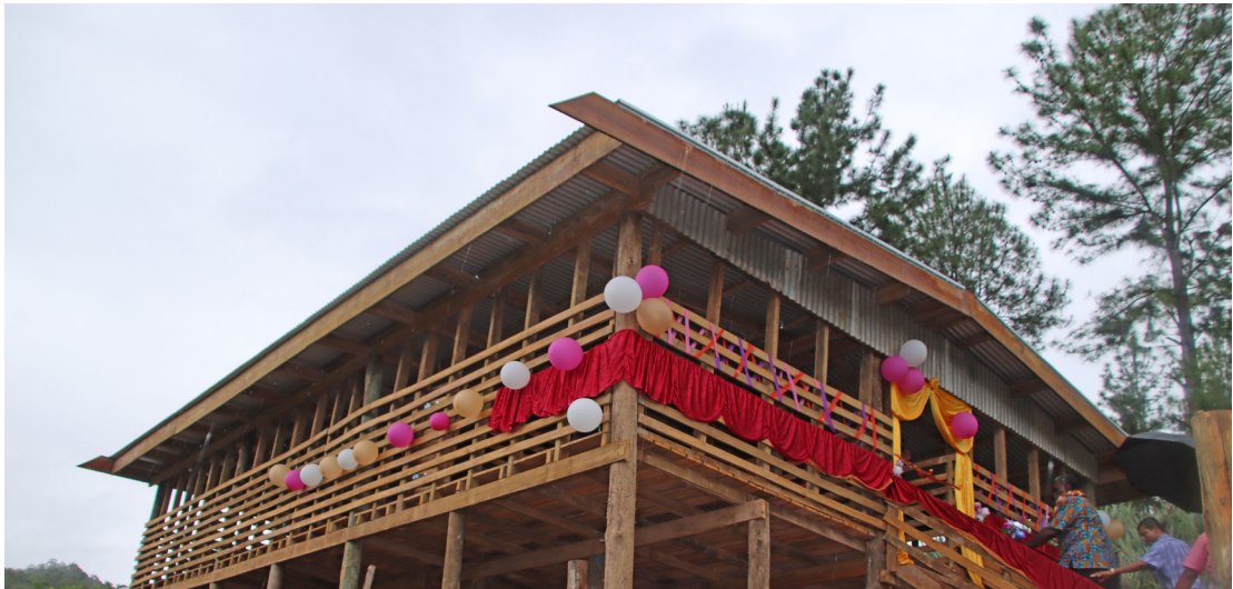
The newly built goat shed belonging to Bhan Pratap.
