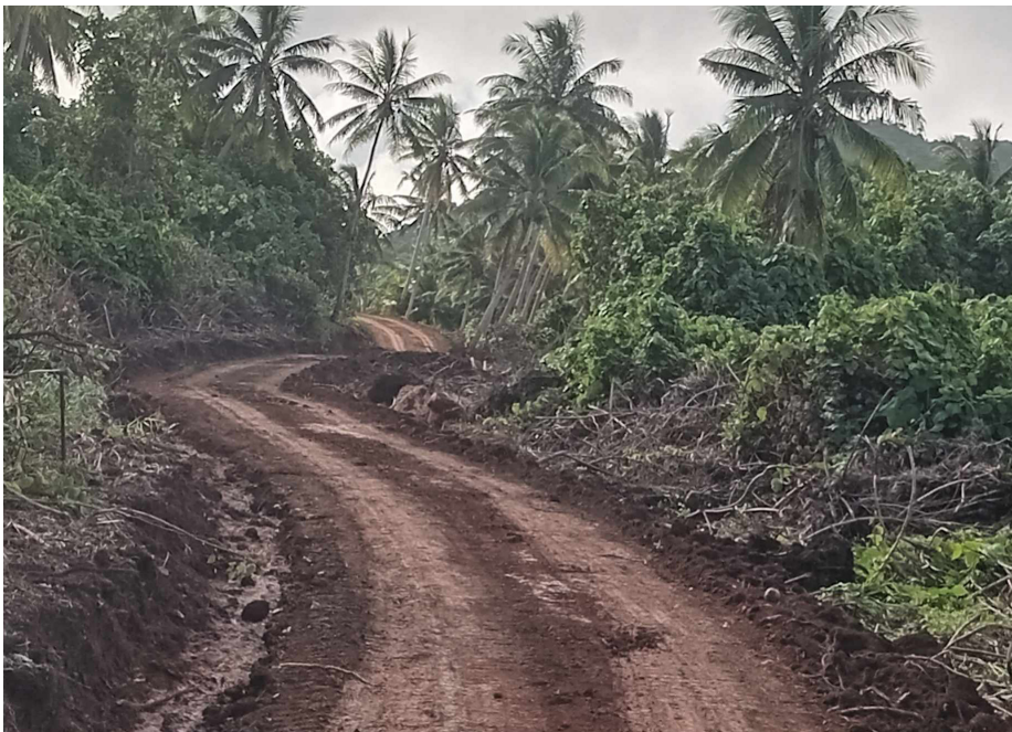
Thirty seven (37) farmers in Vanua Balavu, Lau will now be able to expand their farms and increase their livelihoods after the Ministry of Agriculture and Waterways ongoing farm road construction is fully completed. Photo: SUPPLIED
