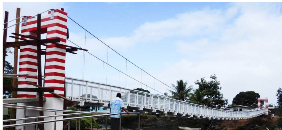
The new suspension bridge in Bua Lomanikoro which was commissioned by Prime Minister, Sitiveni Rabuka recently. Photo: SUPPLIED
