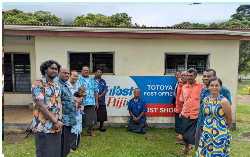
Post Office staff in Totoya, Lau during the installation of solar systems. Photo: POST FIJI
